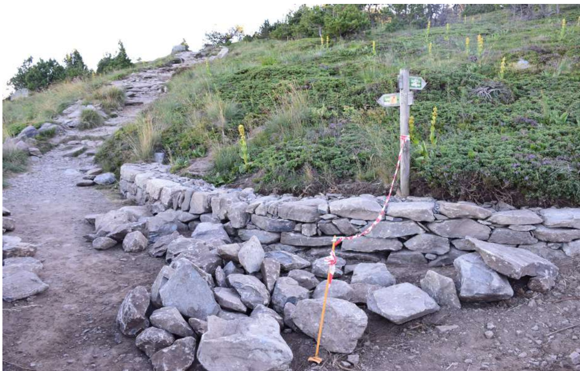
Figure 25. Restoration work on the paths to channel visitors to the Mont Mézenc volcanic geosite (photo N. Klee).
