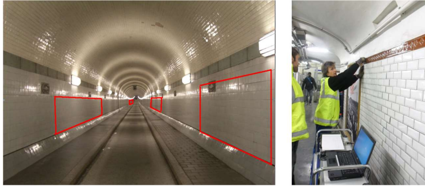
Figure 4. Example of the Meditoss panel inspection
