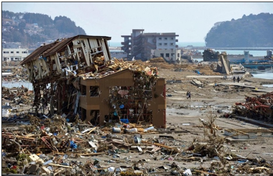
Figure 3.3.2: The coastal town of Minamisanriku in northeastern Japan on March 13, 2011, two days after the tsunami. Destroyed buildings and chaotic deposits, showing mixed debris lying above and inside sediments dumped by the tsunami. © REUTERS/Kyodo, The Atlantic, Alan Taylor, March 13, 2011, 33 photos in focus. ( https://www.theatlantic.com/photo/2011/03/japan-earthquake-aftermath/100023/ )
