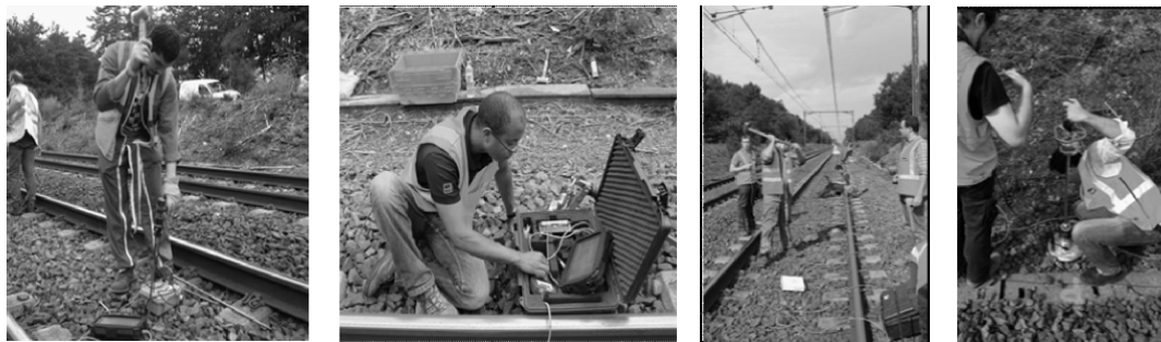
Figure 7: Test campaign carried out on the Vierzon site, (a) Panda 3®, (b) geo-endoscopic tests, (c) MASW and (d) dynamic load plate test [13].
