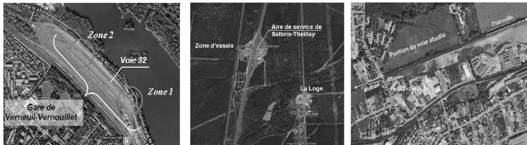
Figure 6: Locations of tested railway sites: (a) Vernouillet (78), (b) Vierzon (18) and (c) Thionville (57) [14].
