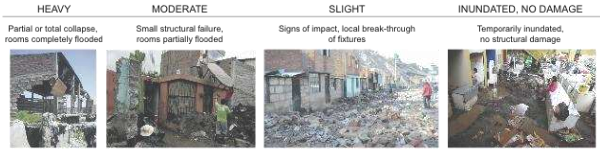
Figure 7: Observed damage levels from left to right (4) inundated, heavy damage, (3) inundated, important damage; (2) inundated, light damage; and (1) inundated, without damage.
